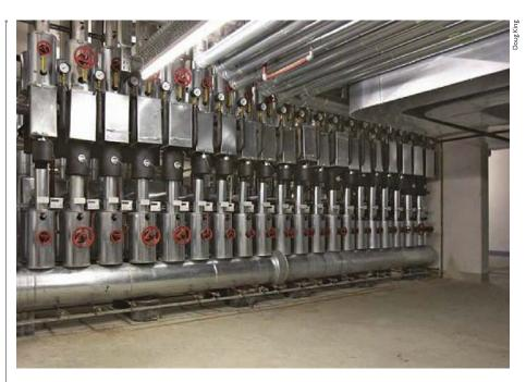
Extensive zoning of heating and cooling systems may lead to more distribution pipework, but it could also create new opportunities to exploit surplus energy from solar or casual gains more easily by maintaining exergy between different parts of the building.
