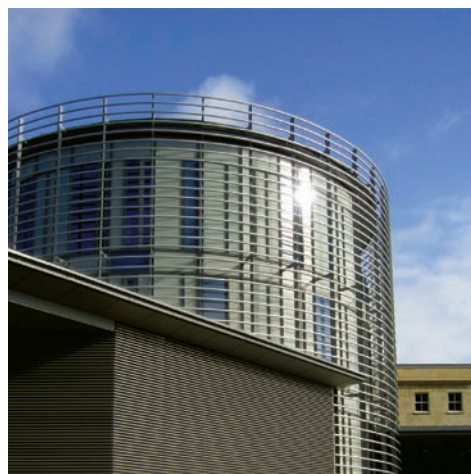
The Ugly Faux brise-soleil on the new Bath Bus Station has minimal effect on heat gains.
