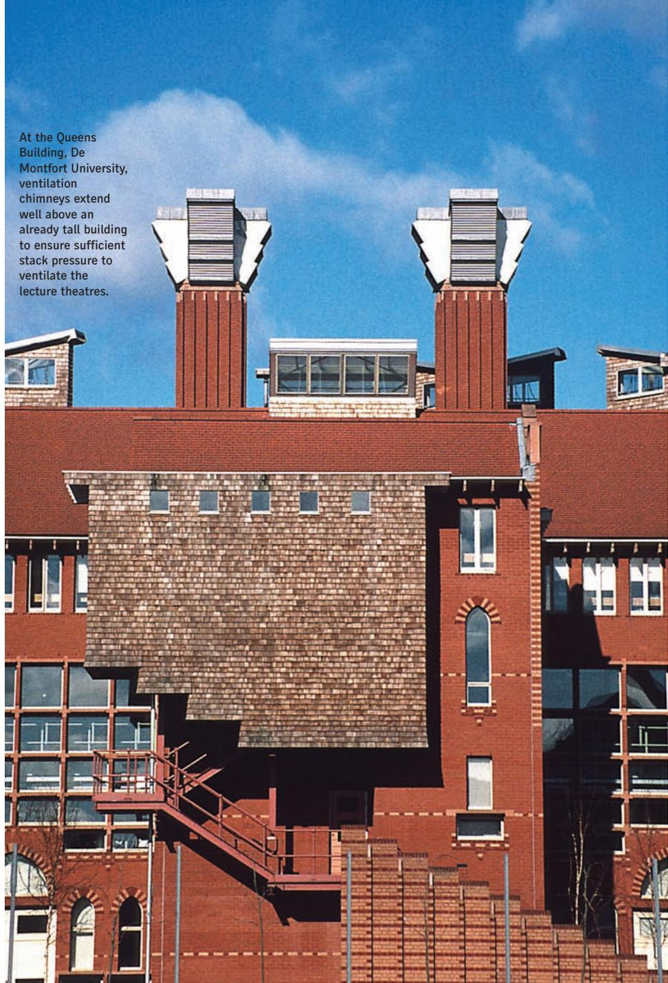
At the Queens Building, De Montfort University, ventilation chimneys extend well above an already tall building to ensure sufficient stack pressure to ventilate the lecture theatres.
